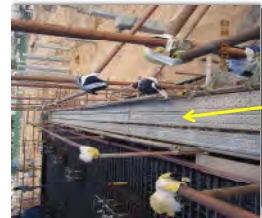
Safe working Platform complete with hand rail, mid rail and toe board
