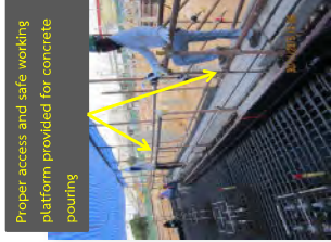
Proper access and safe working platform provided for concrete pouring
